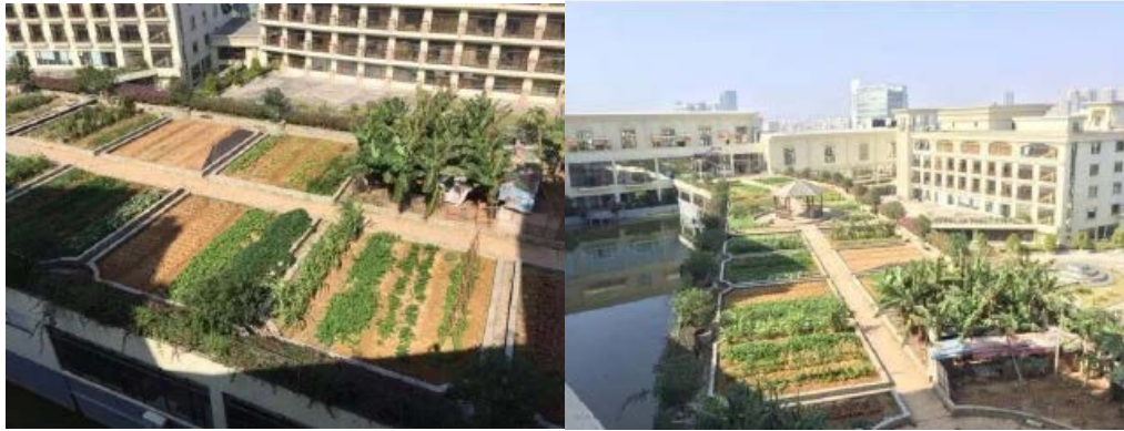
Figure 1. Green Roof Construction Reference Photo Source: Network
